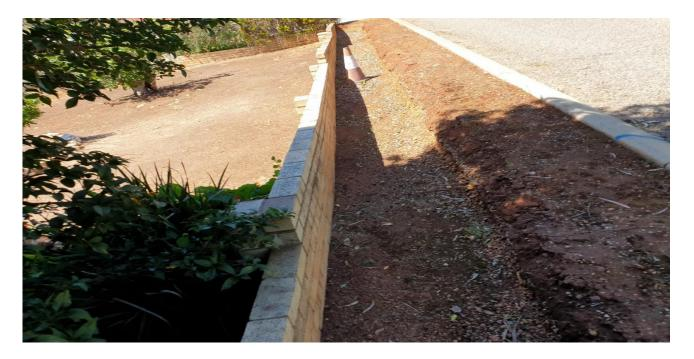
The required action is to replace the single skin brick wall with a retaining wall, and then the backfilling of the trench to provide a safe and single level verge / footpath.
