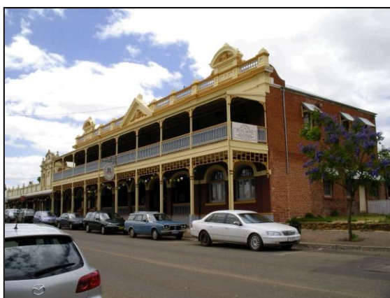
The Freemasons Hotel and Connors Mill provide a good guide to the palette of materials and finishes appropriate to commercial development in the historic town centre
