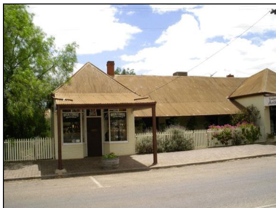
The entry to a shop or other commercial building on Stirling Terrace must be flat and accessible. Any necessary level changes due to the slope of the land can take place inside the building. Front fences and gardens can complement the building behind
