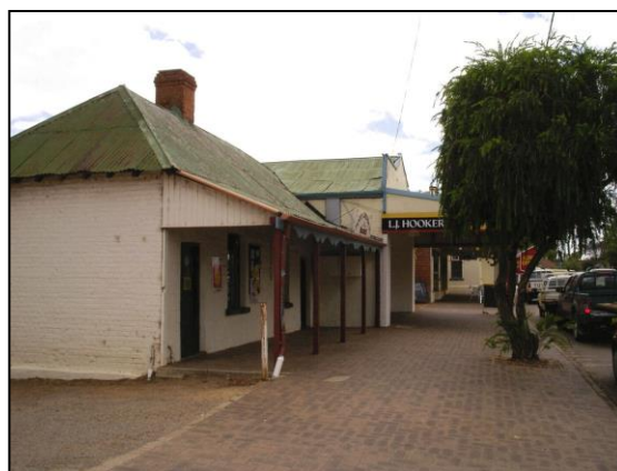
Some existing older buildings have a small front setback to the street
