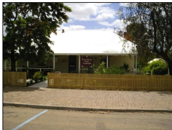
New fencing must be low and constructed of appropriate materials
