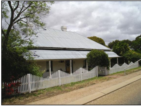
An older dwelling featuring traditional Toodyay building materials
