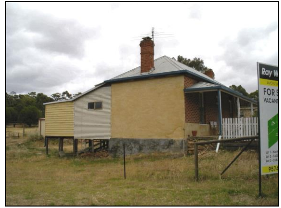
A small cottage with rear extension using a variety of appropriate building materials
