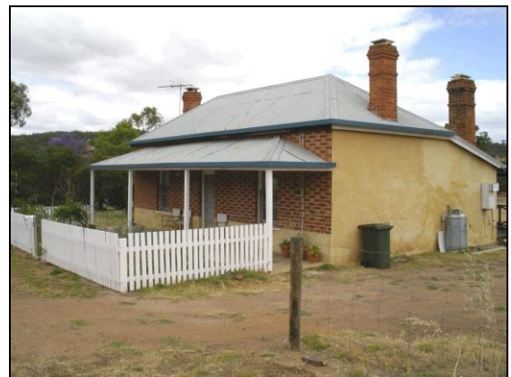
A small cottage with simple roof form, centrally located front door, front verandah and rear extension
