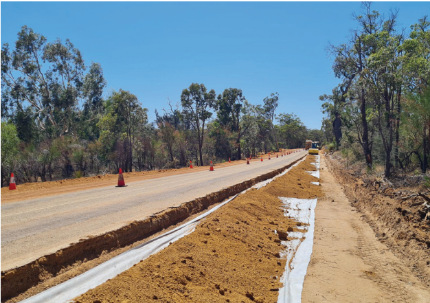
Toodyay Bindi-Bindi Road – Geotextile for soil stabilisation
