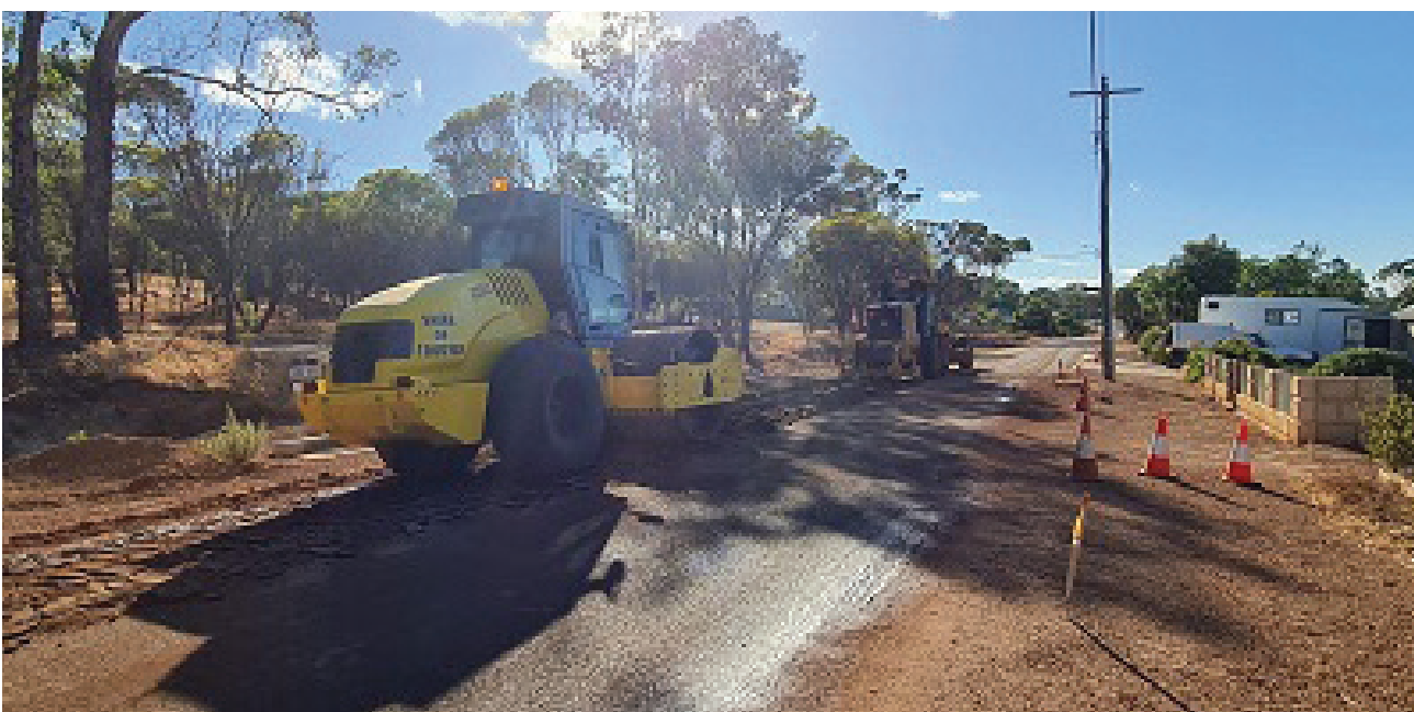
Toodyay Street upgrade – Ripping of existing asphalt
