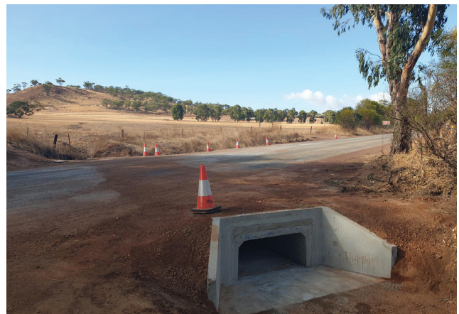
Completed culvert crossing and headwall.
