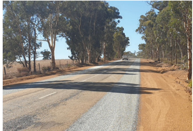
Completed shoulder widening and sealing
